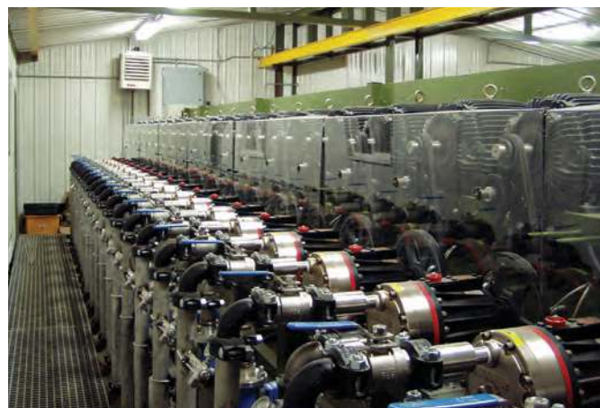
Hydra-Cell pumping shear-sensitive polymers for enhanced oil recovery.
