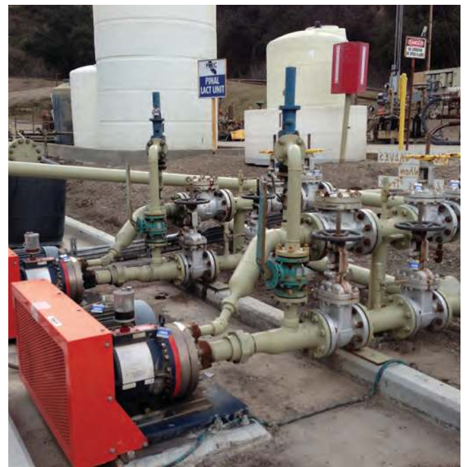
Hydra-Cell pumps shown processing volatile crude oil.
