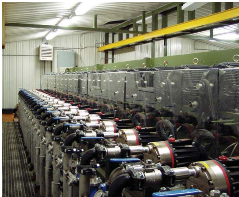
Figure 1. Polymer injection plant designed and built by FabTech, incorporating 21 seal-less Hydra-Cell H25 pumps.
