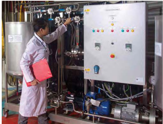
RO treatment of waste streams at a pharmaceutical processing facility.
