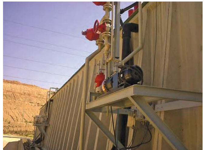
Long-distance transfer to a water and wastewater treatment plant.
